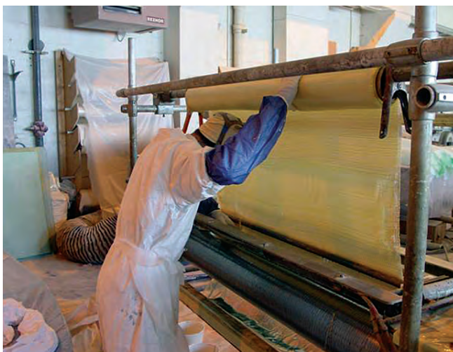
(From top) Peel ply and breather are placed over the laminate before the vacuum bag is applied; Kevlar is applied to the hull sides for added impact resistance; BBW's impregnator wets out the fiberglass reinforcement to a precise 60/40 glass-to-resin ratio, the opposite ratio found in many open-molded boats.
